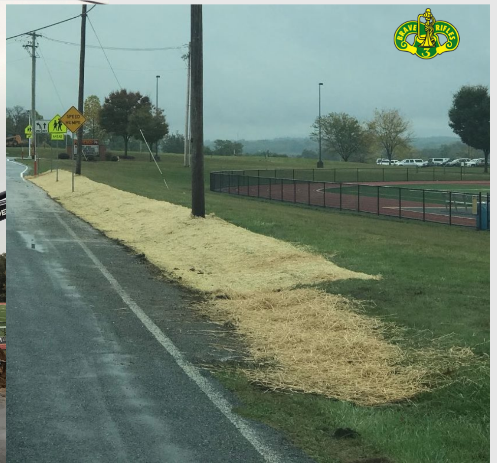
Drainage Fix Ped Safety Grant
